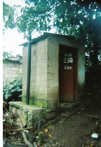
**FIGURE 4** | An example of picture linking participants' feeling with infrastructures. Exterior view of a "Ventilated Pit Latrine" (VIP) in Dassenveld (South Africa). The pipe on the left of the structures helps to remove odor from inside the latrine. "That's the toilette, this is the outside...there is no lock." Credits: 34 year old woman, Photovoice project, Source: Scorgie.
